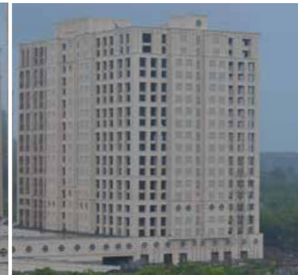
NEWCASTLE - EXTERIOR FACADE FINISHING WORK NEAR COMPLETION
