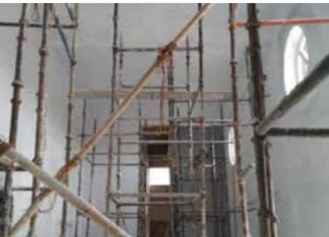
ATLAS - PANEL ROOM WHITEWASH WORK IN PROGRESS
