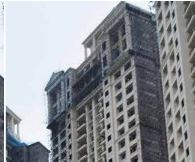
MELLONA - EXTERNAL FACADE PAINTING IN PROGRESS
