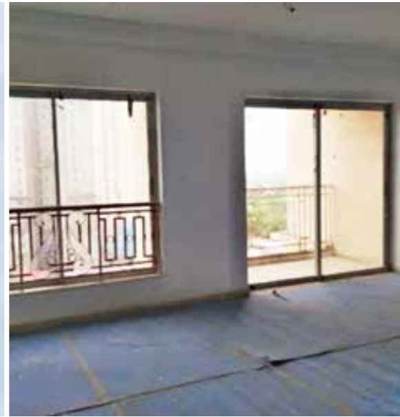
FIXING OF WINDOWS SHUTTER IN PROGRESS IN VARIOUS BUILDINGS
