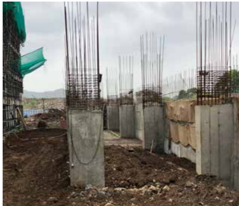
SECTOR C - RETAINING WALL WORK IN PROGRESS
