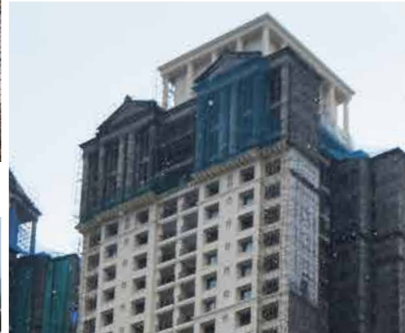
CLIO - EXTERNAL FACADE PAINTING IN PROGRESS
