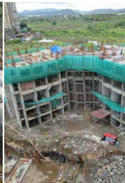
ZEUS - LEVEL 4 SLAB COMPLETED
