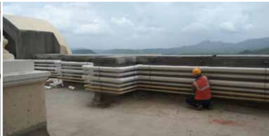
ATLAS - LOOPING WORK AT TERRACE IN PROGRESS
