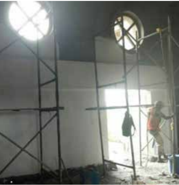
HELIOS - PANEL ROOM WHITEWASH WORK IN PROGRESS
