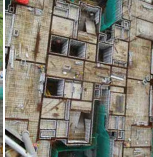
ORION - LEVEL 4 SLAB COMPLETED
