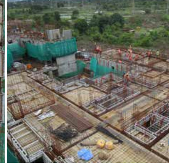
SELENE - LEVEL 4 SLAB COMPLETED
