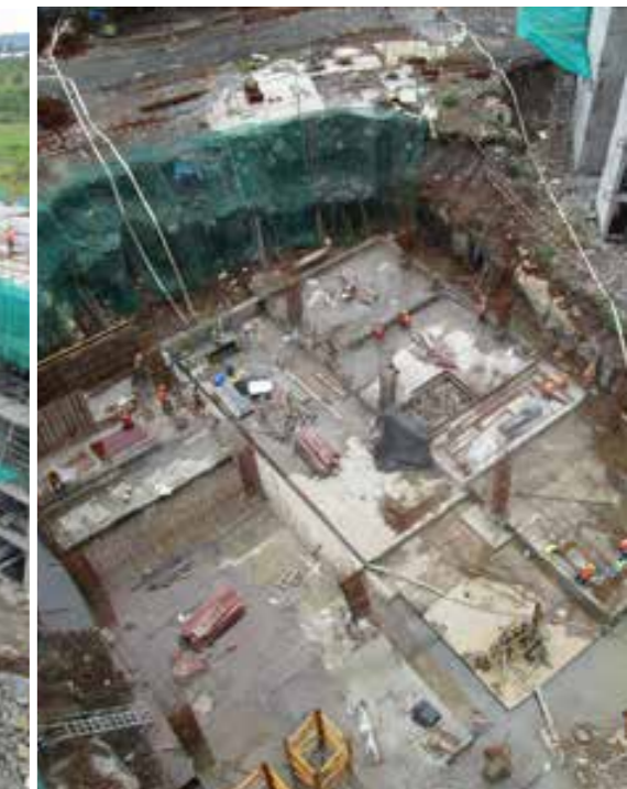
SECTOR C - UG WATER TANK NO. 1 CONSTRUCTION IN PROGRESS
