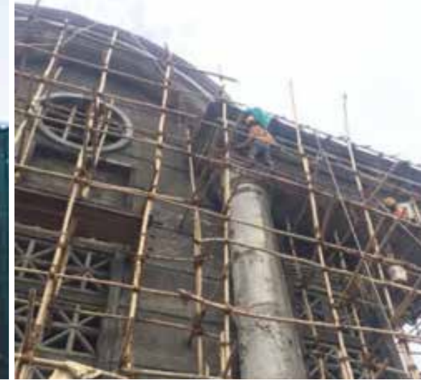
ARGUS - PLASTER WORK ABOVE TERRACE IN PROGRESS
