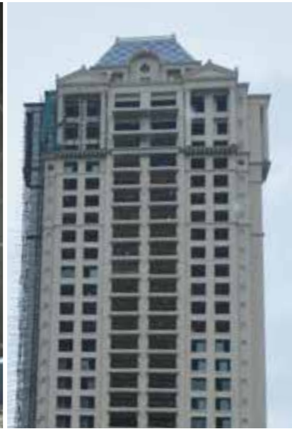
HERMES - EXTERNAL FACADE PAINTING IN PROGRESS
