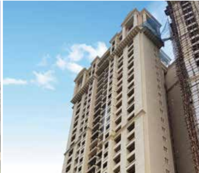
ATLAS - EXTERNAL FACADE PAINTING IN PROGRESS
