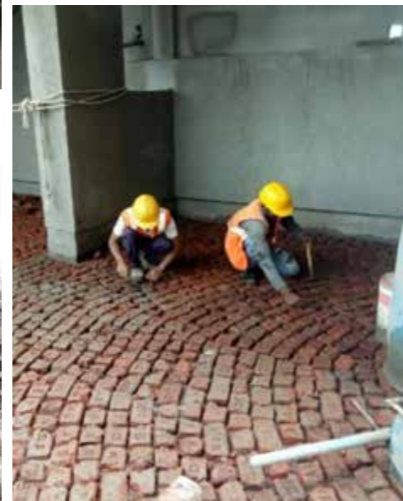
MELLONA - TERRACE WATERPROOFING WORK IN PROGRESS
