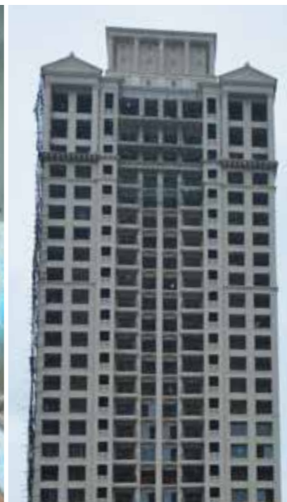
HELIOS - EXTERNAL FACADE PAINTING IN PROGRESS
