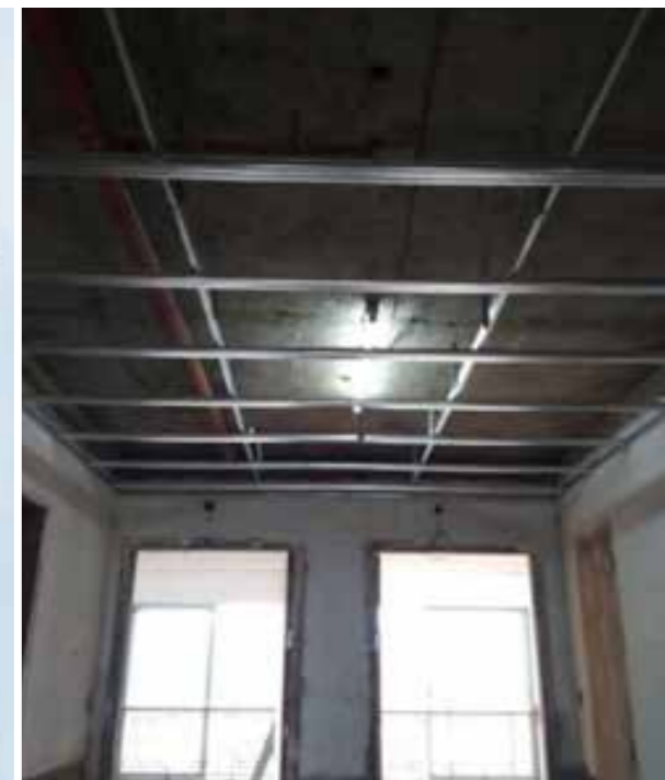
HELIOS - CEILING WORK AT LOBBY IN PROGRESS
