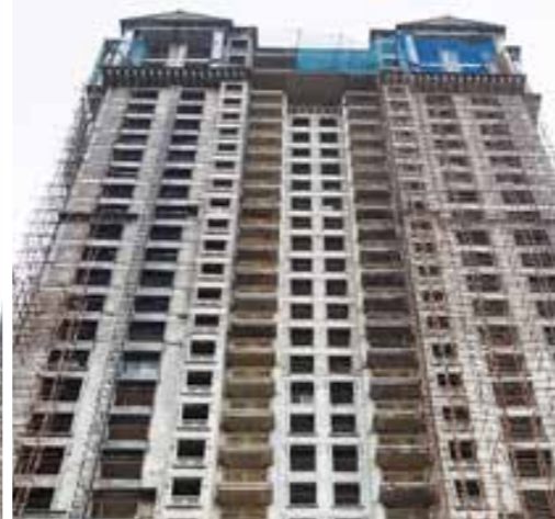
AURA - EXTERNAL FACADE PAINTING IN PROGRESS
