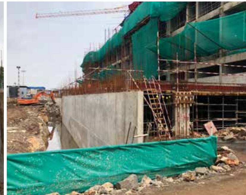
SECTOR C - RETAIL AREA CONSTRUCTION IN PROGRESS
