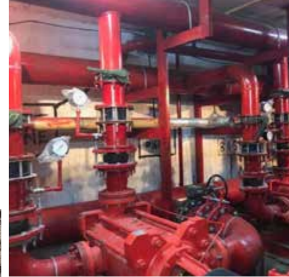
AURA - PUMP ROOM FITTING NEAR COMPLETION
