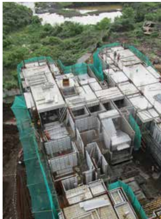
VENUS - LEVEL 4 SLAB COMPLETED
