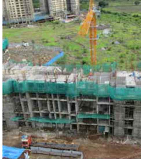
HERA & VESTA - LEVEL 4 SLAB COMPLETED
