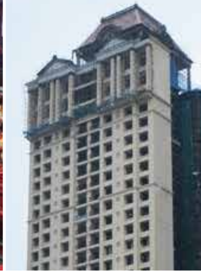
ARGUS - EXTERNAL FACADE PAINTING IN PROGRESS
