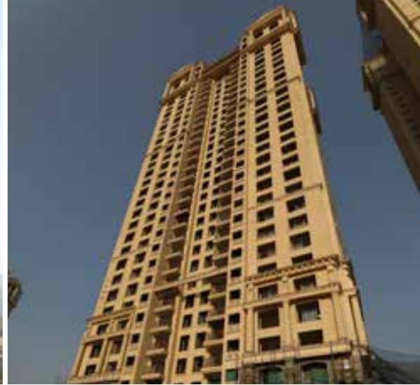
AURA: CONSTRUCTION IN FULL SWING
