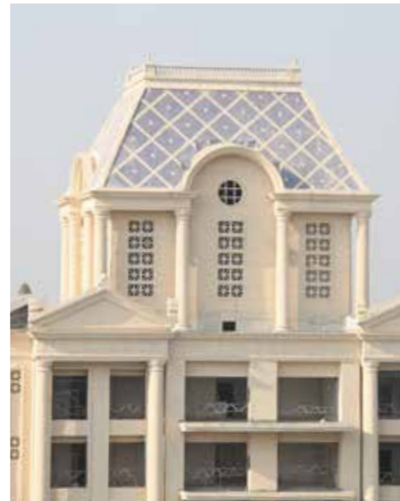
HERMES: DOME PAINTING HAS BEEN COMPLETED
