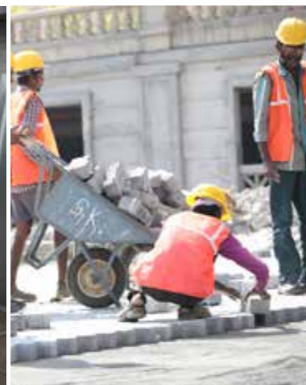
PAVER TILES FIXING AT RAMP 2 FOR VEHICULAR TRAFFIC
