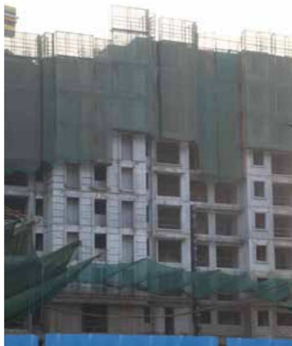
HERA & VESTA: CONSTRUCTION IN PROGRESS
