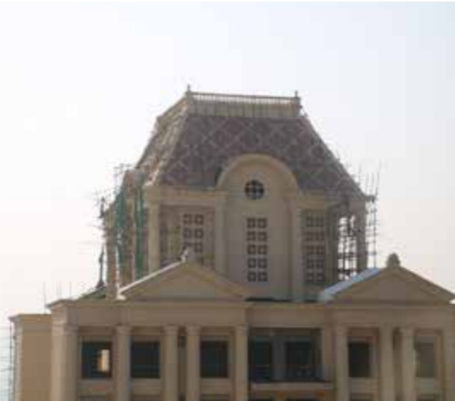
ARGUS: PAINTING OF THE DOME NEARING COMPLETION
