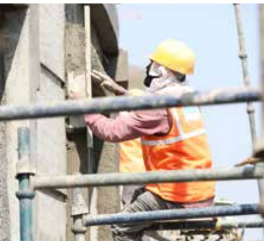
AURA: PLASTERING WORK IN PROGRESS
