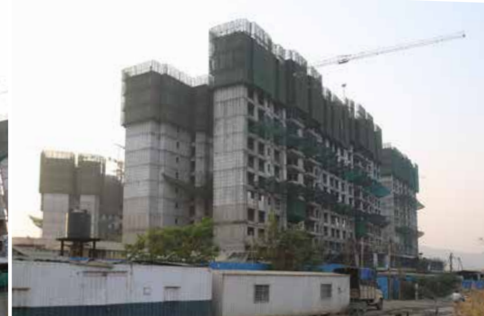
FLORA & SELENE: CONSTRUCTION IN PROGRESS
