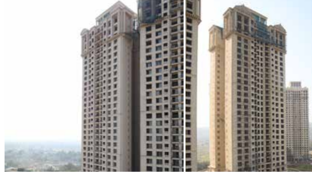
ATLAS: EXTERNAL PAINTING NEARING COMPLETION
