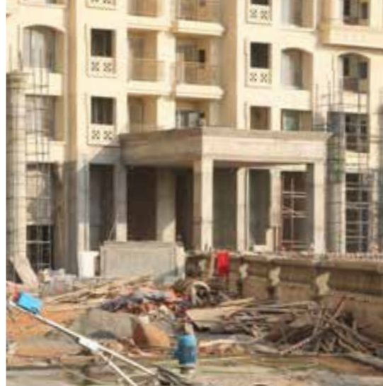
ATLAS: PODIUM ROAD CONSTRUCTION IN PROGRESS
