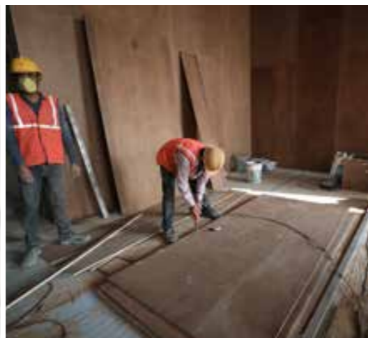
AURORA: ENTRANCE LOBBY WORK IN PROGRESS
