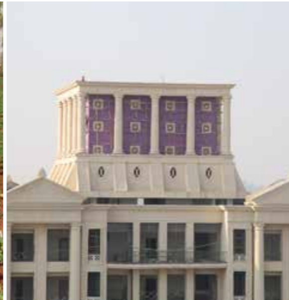
MELLONA: DOME PAINTING HAS BEEN COMPLETED
