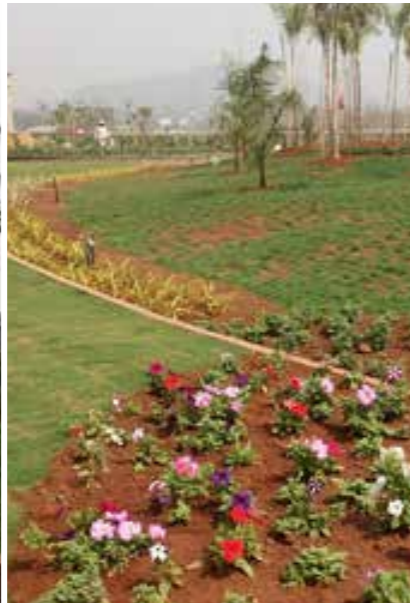
LANDSCAPING WORK OF PODIUM GARDEN - A IN PROGRESS
