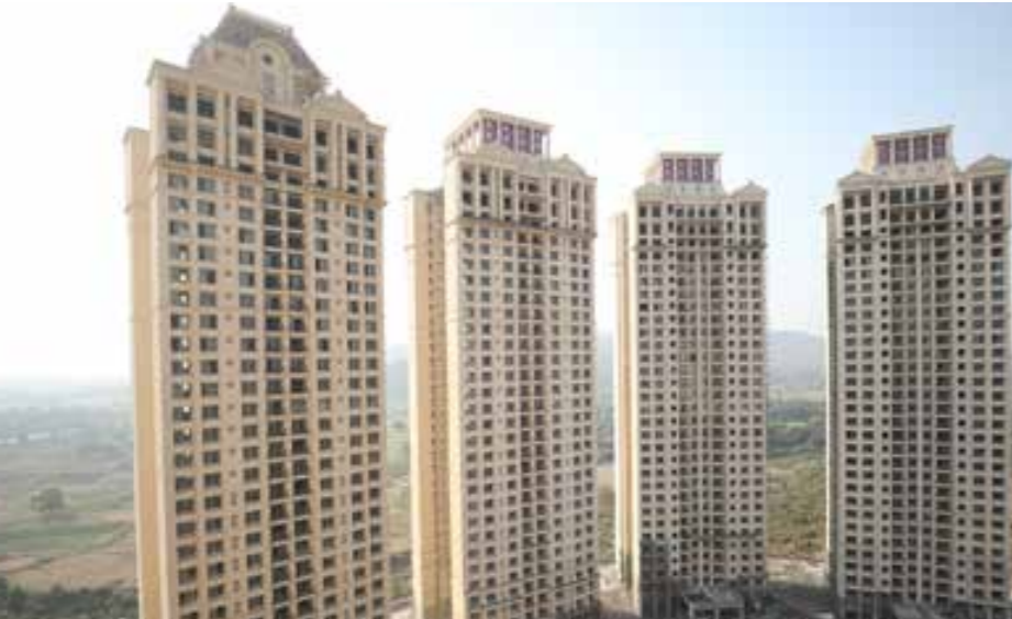
ARGUS, CLIO, MELLONA, HELIOS: EXTERNAL PAINTING NEARING COMPLETION
