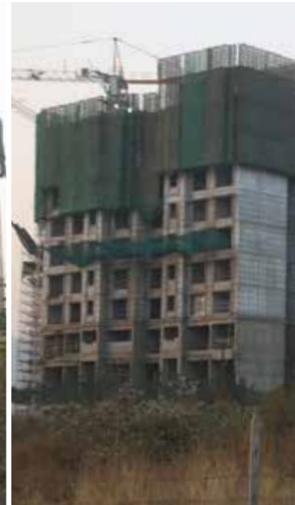
ZEUS: CONSTRUCTION IN PROGRESS
