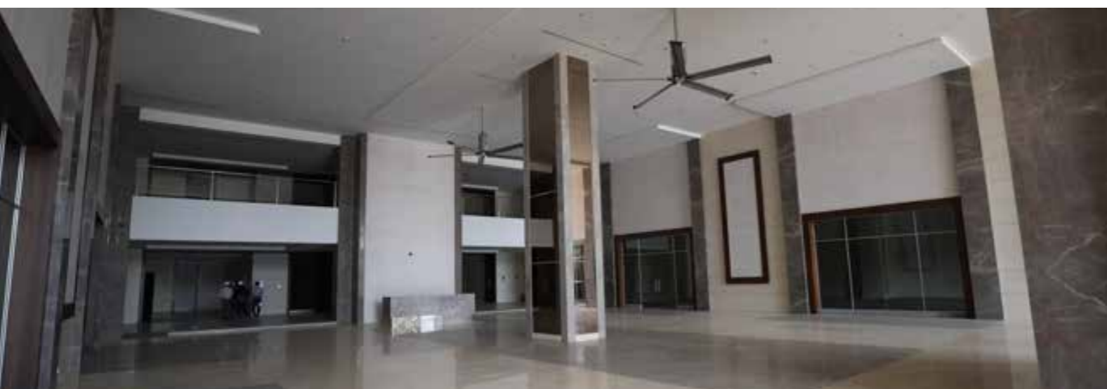
EDINBURGH: LOBBY CONSTRUCTION NEARING COMPLETION
