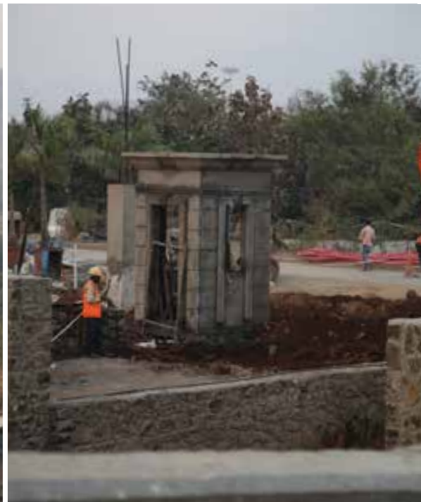
ENTRANCE TO PODIUM UNDER CONSTRUCTION
