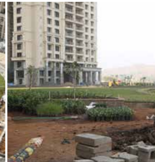
PODIUM GARDEN LANDSCAPING IN PROGRESS
