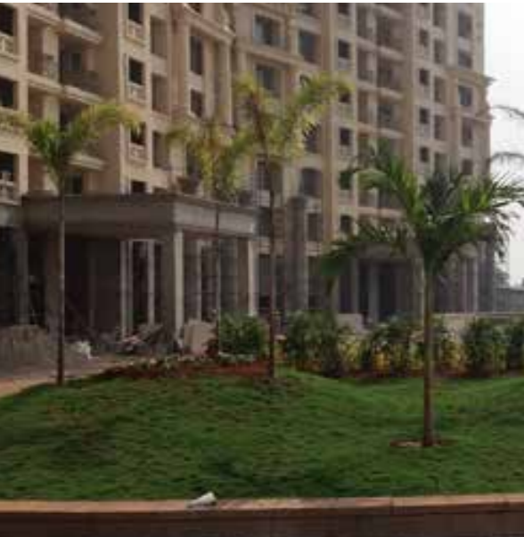
LANDSCAPING WORK OF PODIUM GARDEN - B IN PROGRESS
