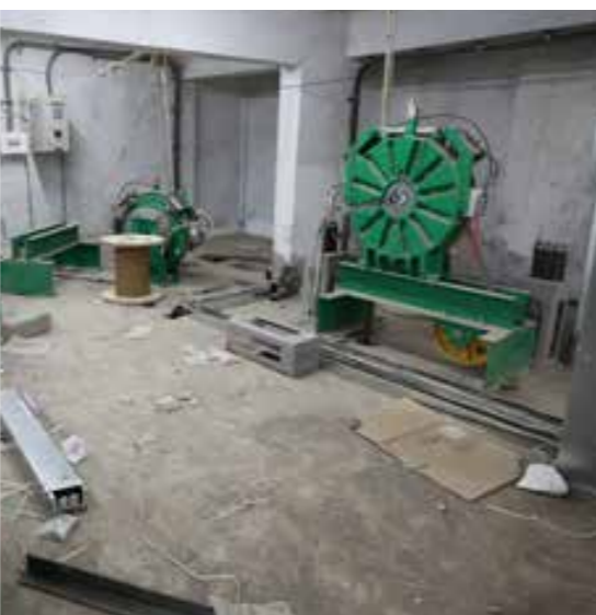
HERMES: LIFT MACHINERY INSTALLATION IN PROGRESS
