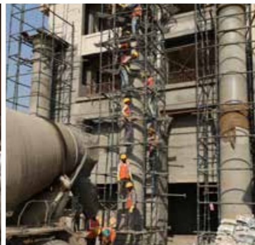
NEO-CLASSICAL FINISHING IN PROGRESS
