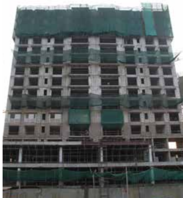
ARTEMIS: CONSTRUCTION IN PROGRESS
