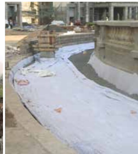
GEO-TEXTILE SHEET FIXING PRIOR TO LANDSCAPING
