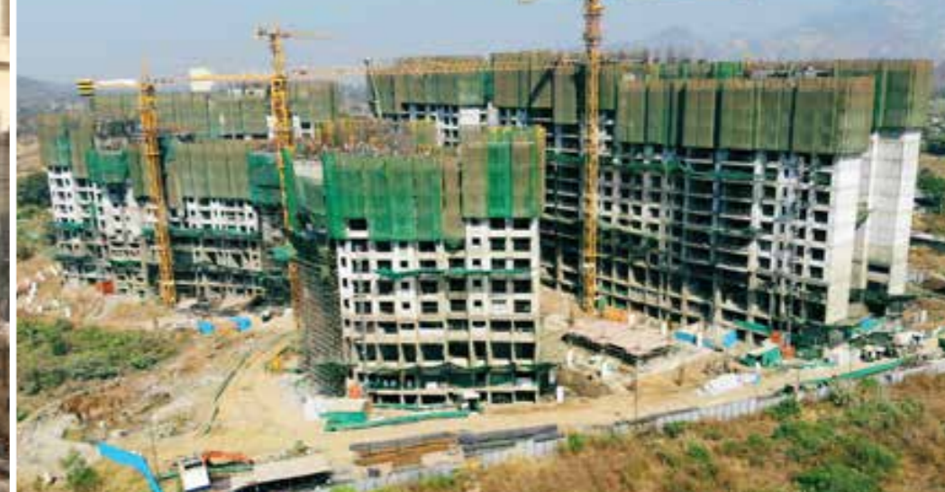
ARTEMIS, HERA, FLORA, VESTA, VENUS, SELENE, ORION, ZEUS: CONSTRUCTION IN PROGRESS
