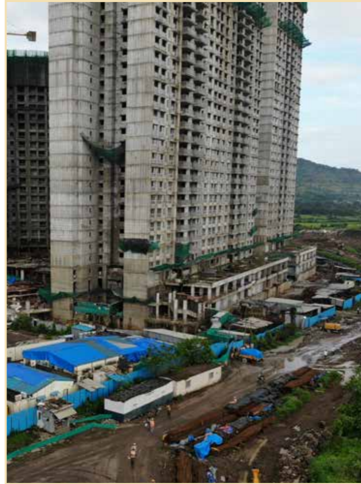
Project Flora: Construction work in full swing
