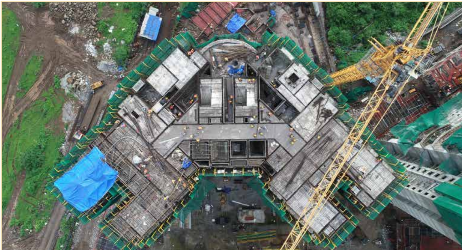
Project Zeus: Construction work in full swing
