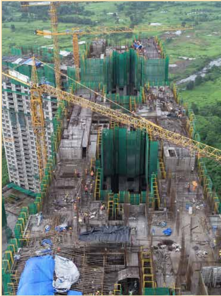
Projects Flora, Selene and Artemis: Construction work in full swing
