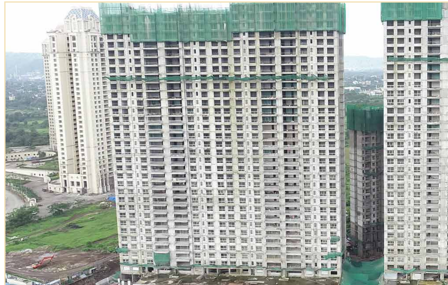
Projects Flora and Selene: Slab 28 and 29 have been completed respectively
