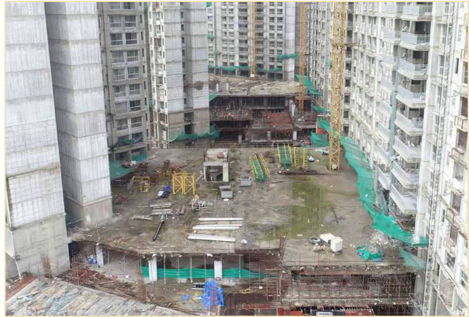
Podium construction work in full swing
