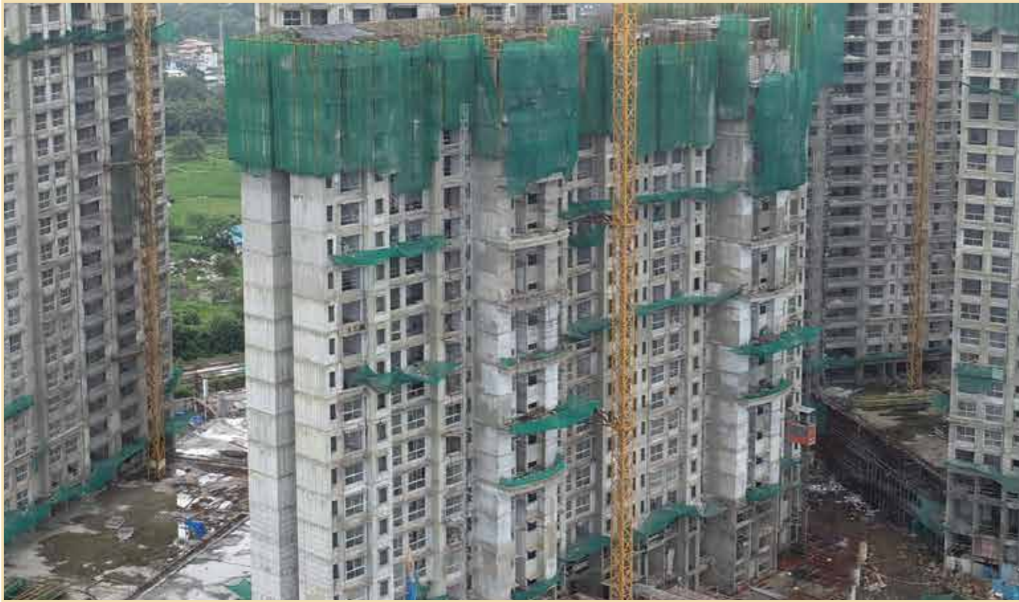
Projects Hera and Vesta: Slab 22 and 20 have been completed respectively
