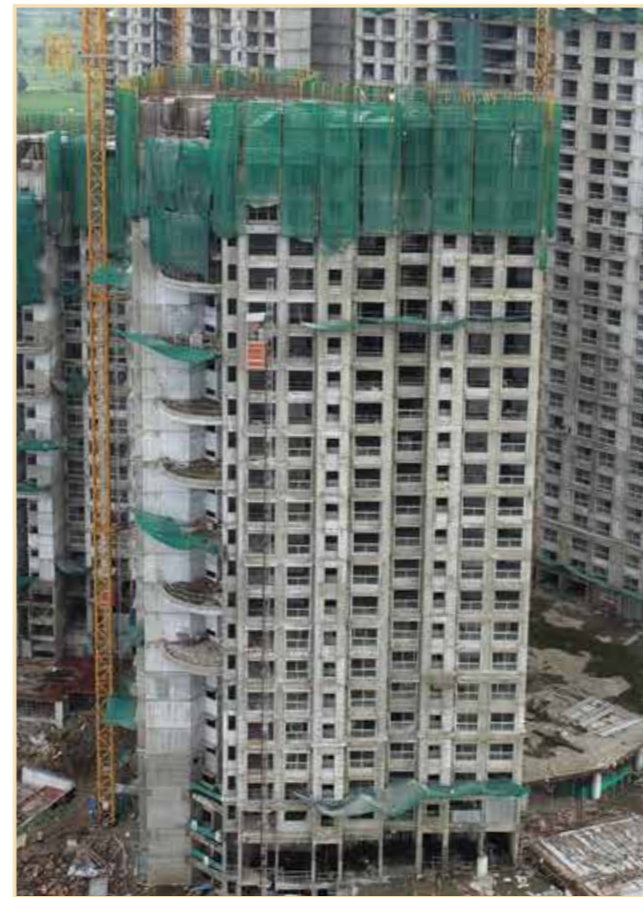
Project Zeus: Slab 25 has been completed
