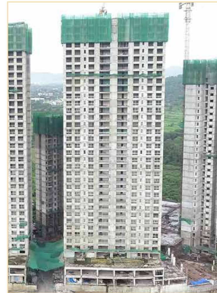
Project Artemis: Slab 30 has been completed
