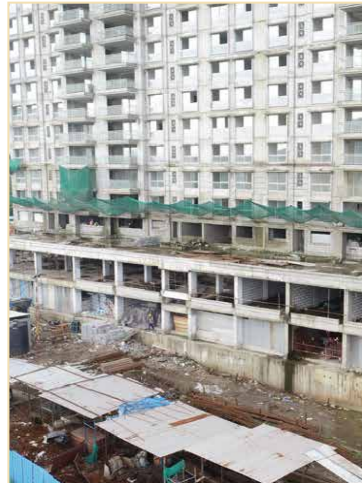
Retail area under construction
