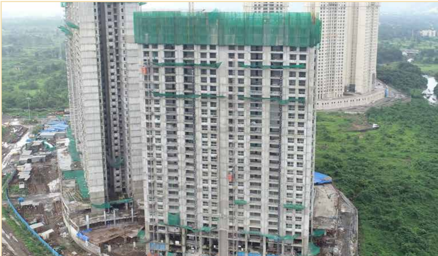
Projects Venus and Orion: Slab 28 and 29 have been completed respectively
