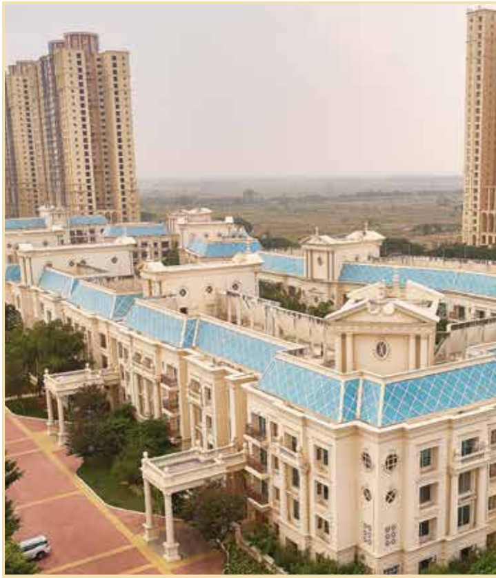
Cluster view of our low-rise buildings, with The Highlands, South in the background
