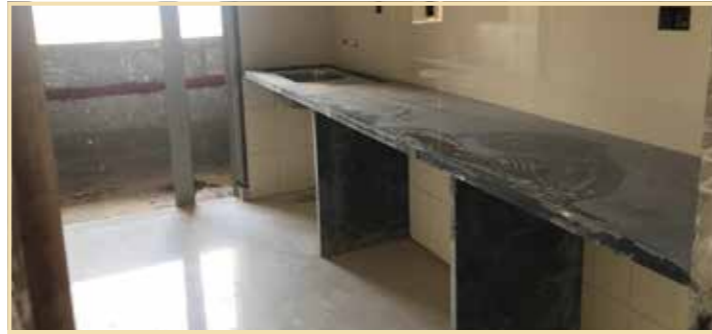
The Highlands South, Warwick I & II: Kitchen finishing work in progress
