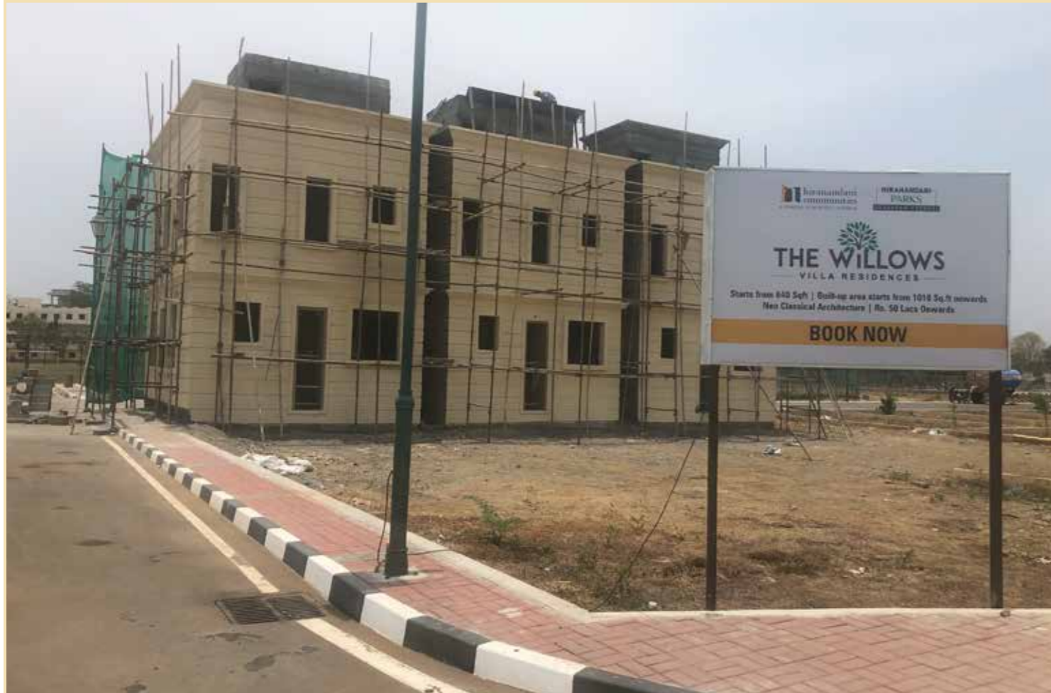
Rear elevation of The Willows: finishing work in progress
