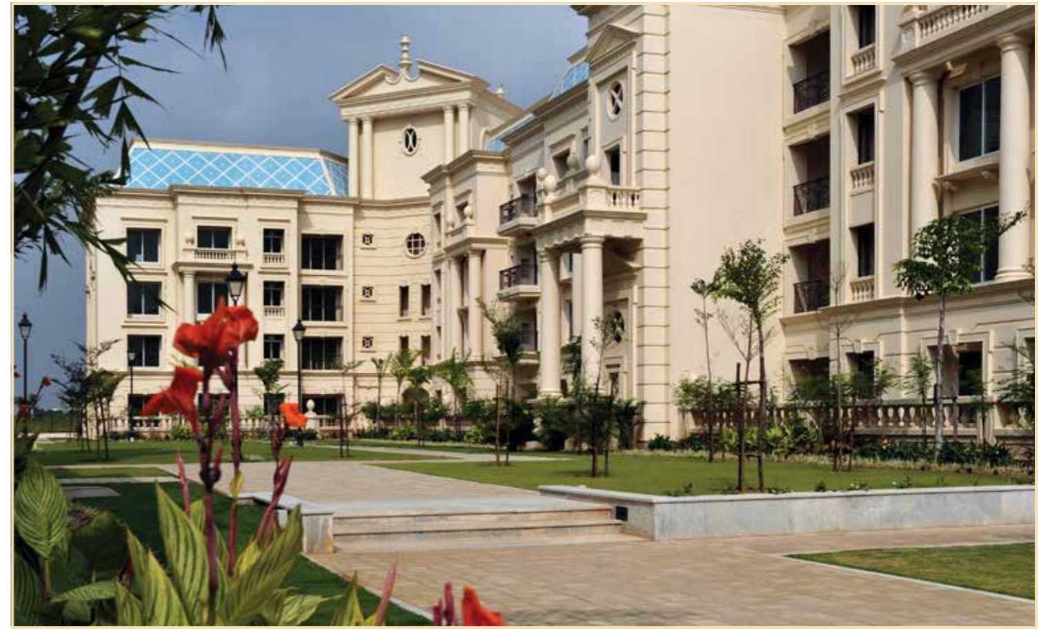
Landscaped garden within the low-rise buildings cluster
