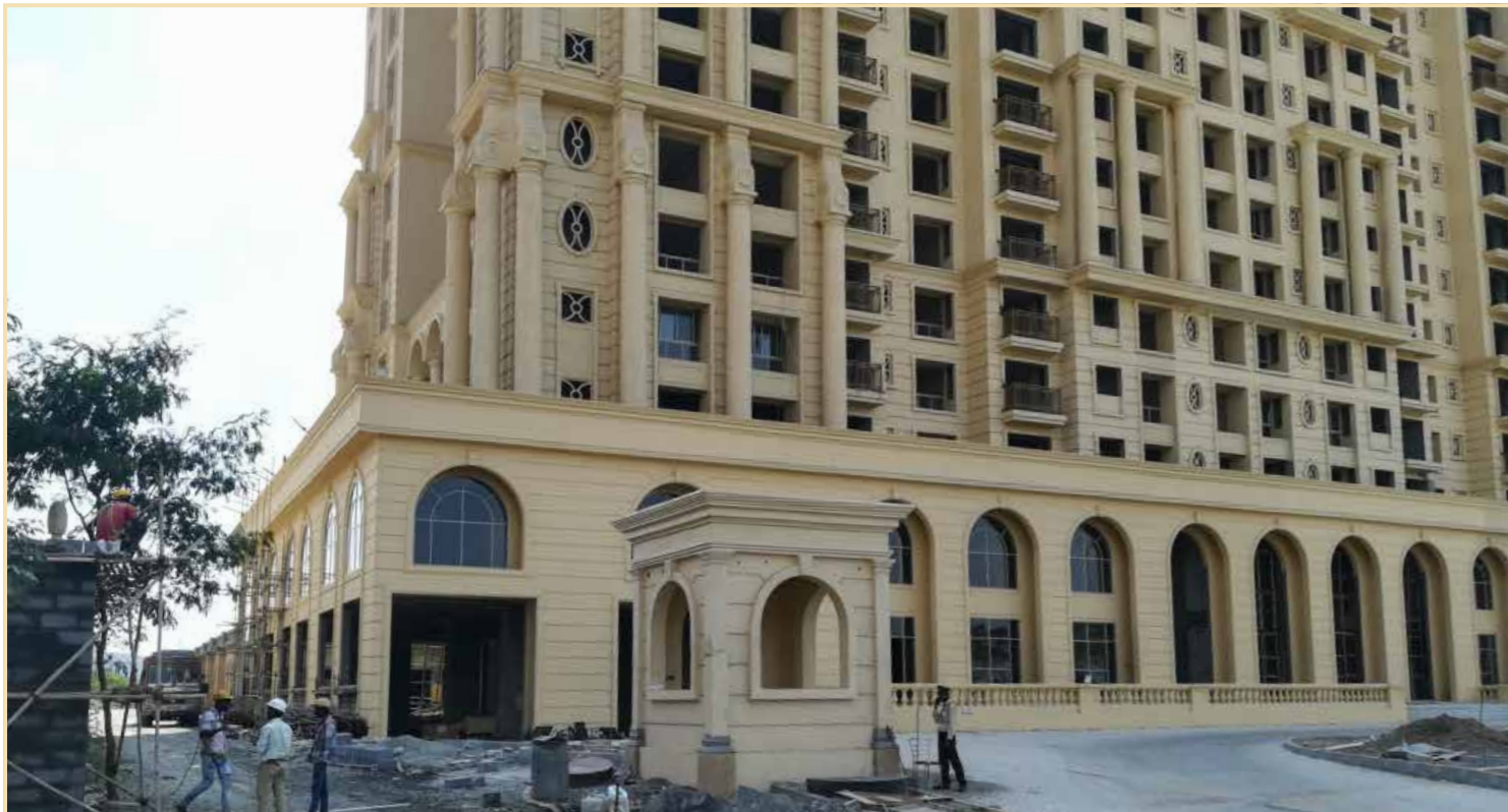
The Highlands South, Chatsworth I & II: Security cabin construction in progress
