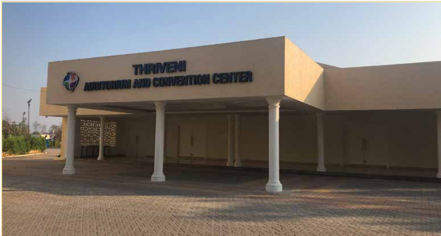
Thriveni Auditorium: facade is completed
