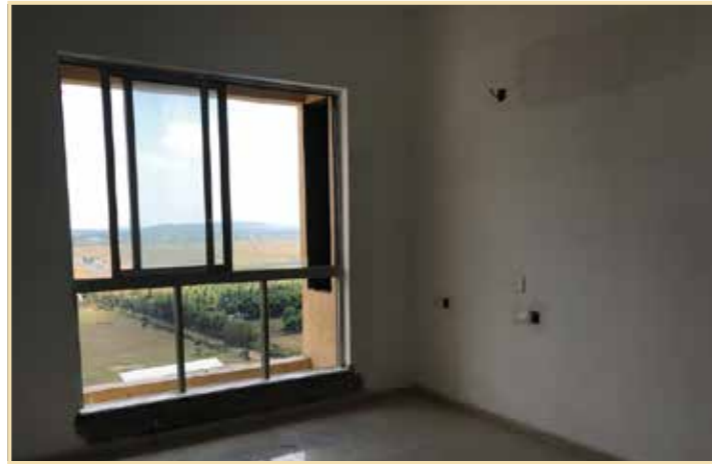
The Highlands South, Warwick I & II: Bedroom finishing work in progress
