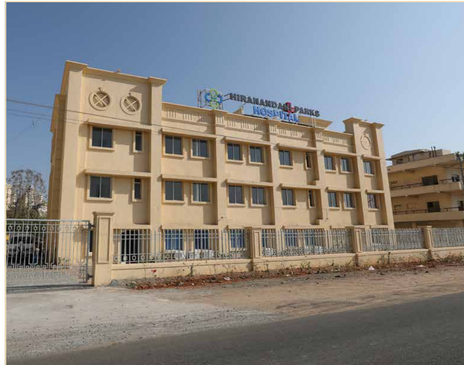
Facade view and entry from Thriveni road for Hiranandani Parks Hospital
