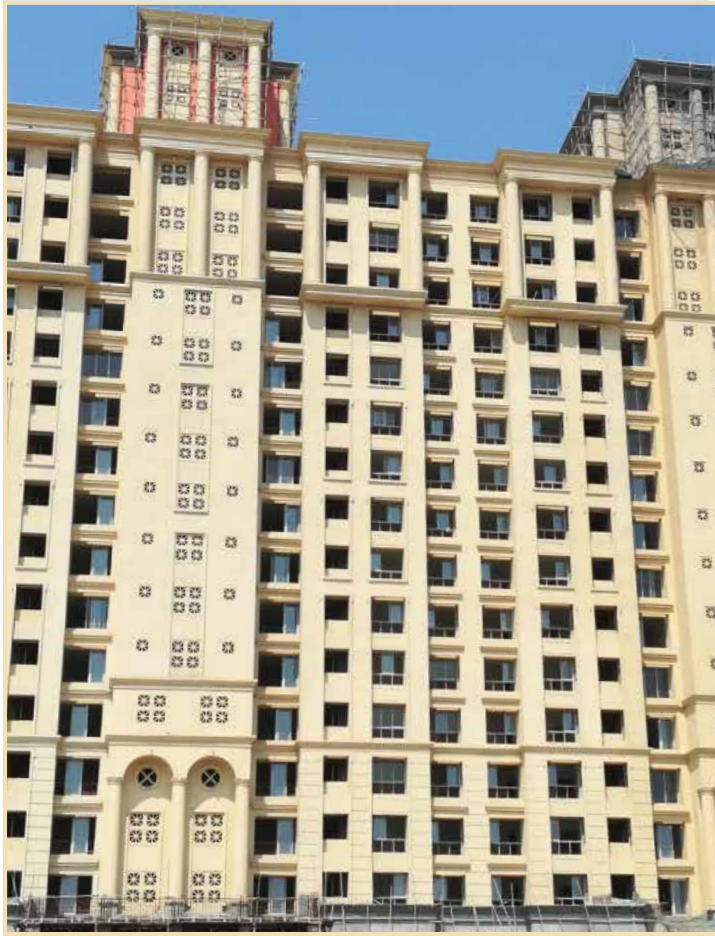
The Highlands South, Warwick I & II: Front facade work in progress
