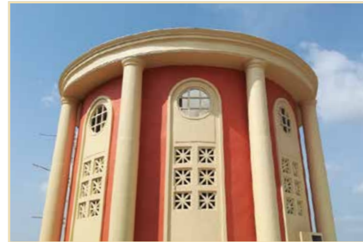
The Highlands South, Chartwell I & II: Life maintenance room and terrace finishing work in progress
